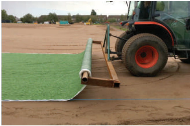
Carpet-hybrid pitch being laid at Thatto
