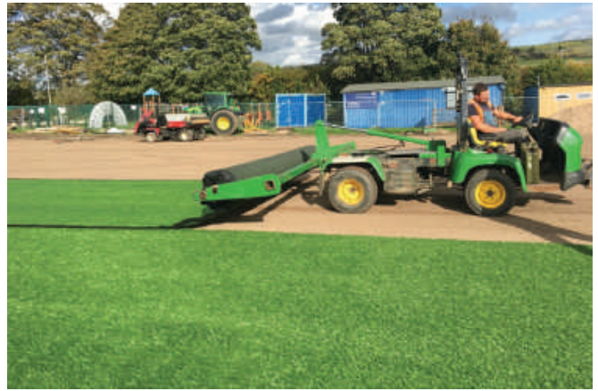
Siddal's carpet-hybrid installation under way
